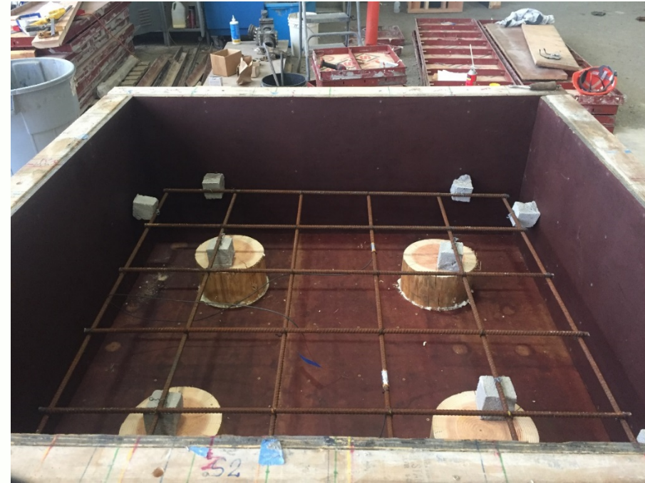
Typical Timber Pile Footing
